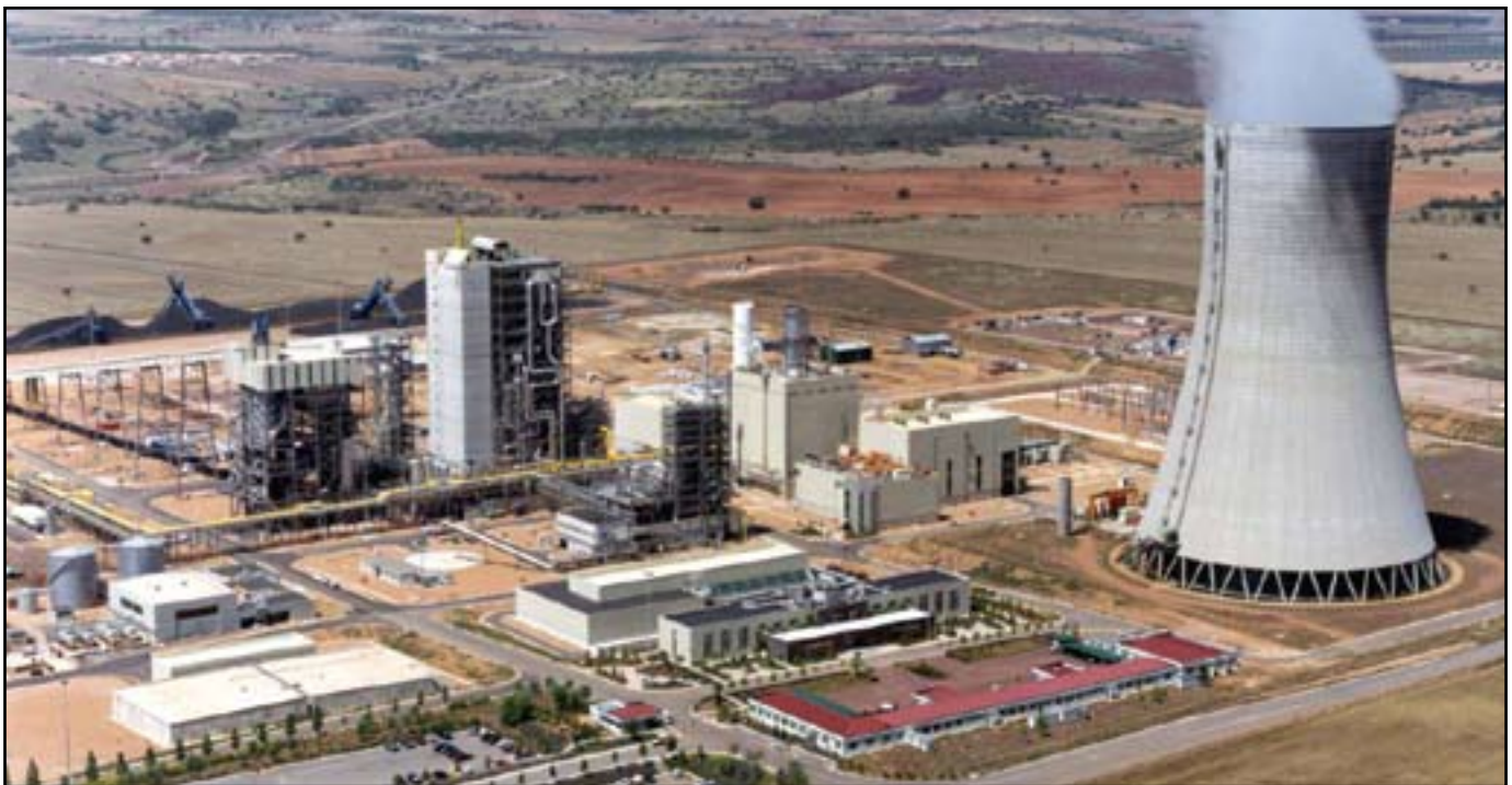
300 MW Puertollano IGCC plant. Coal-based plant will have completed 10 years of commercial gasification operation in March 2008. Powered by a Siemens syngas-modified V94.3 gas turbine power block fed by a gasified mix of petroleum coke and low-grade coal (40% ash) feedstock. Industry's current commercial IGCC plant offerings are powered by F-technology gas turbines.
